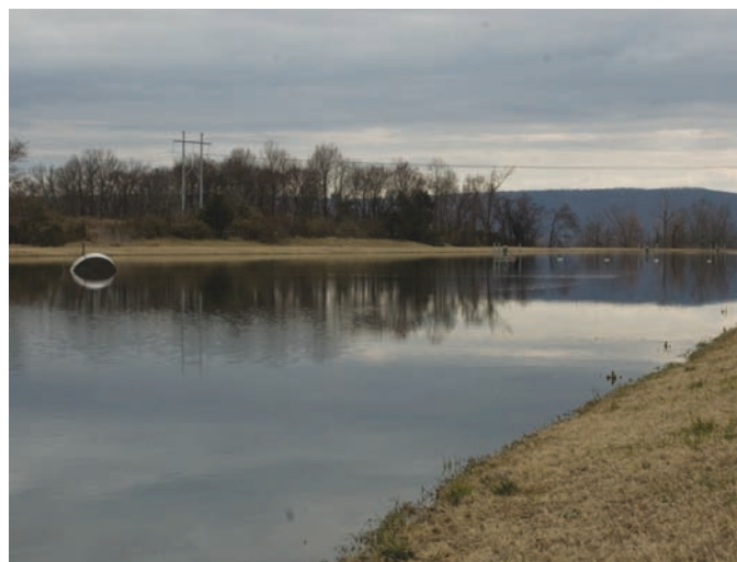
Atkins must wait for drier weather before it can repair tornado-damaged units at its sewer treatment facility.
