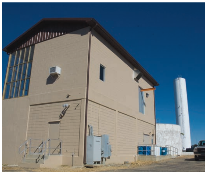
With just a bit of trim work left to do, Dierks' new water treatment plant is again serving the community after being reduced to rubble.
