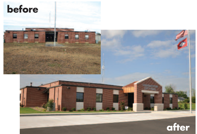
Charleston in just six months converted the former National Guard armory into the city's new municipal complex.
