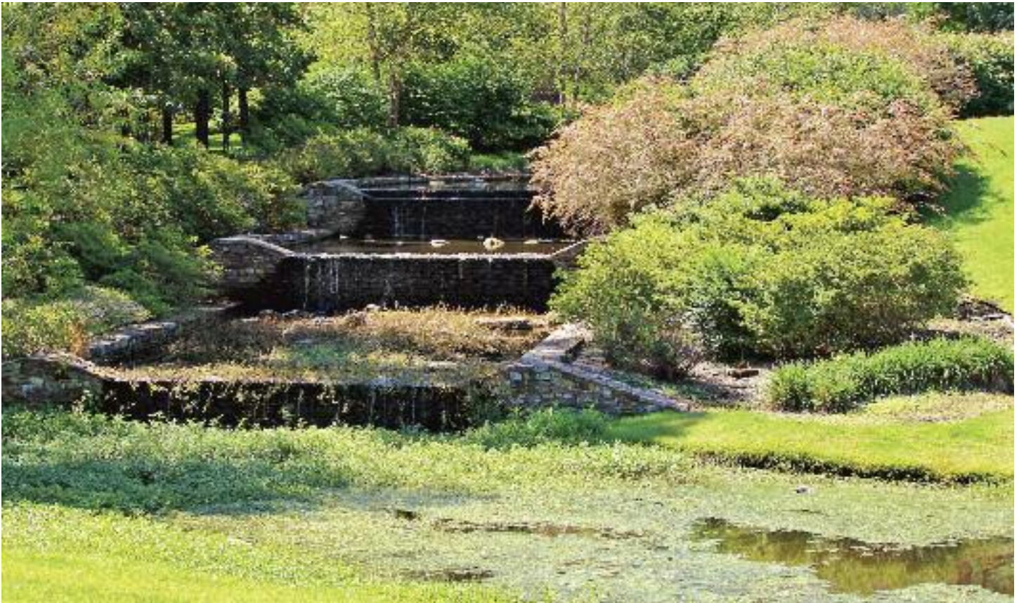
This swale with rock weirs helps solve drainage issues in west Little Rock.
