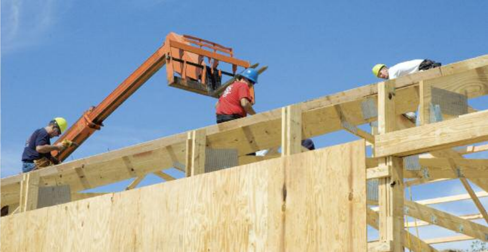
Workers frame the roof of Mena's new 4-H community center.
