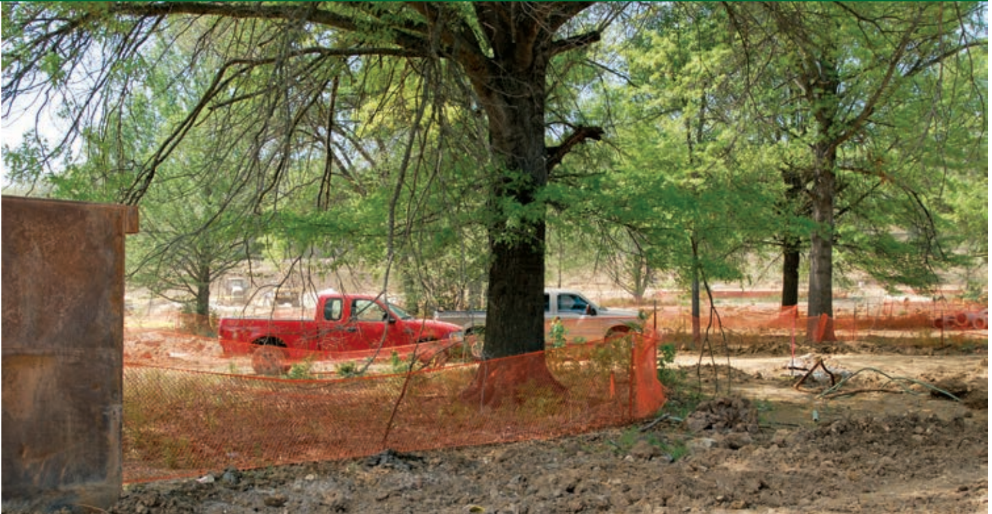
Mature trees on construction sites need more protection, especially in their critical root zones.
