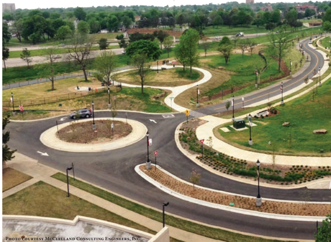
PHOTO COURTESY MCCLELLAND CONSULTING ENGINEERS, INC.
