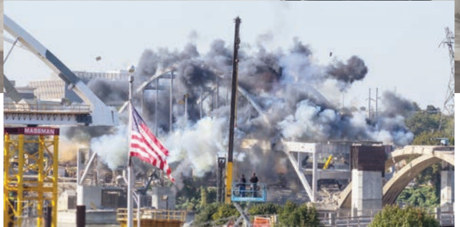
It took several rounds of implosions and some additional pulling by tugboats to bring down the old bridge. The steel span and structural upgrades to the bridge made in 1974 proved more difficult to demolish than the original, concrete portions of the bridge, which dated back to 1923.
