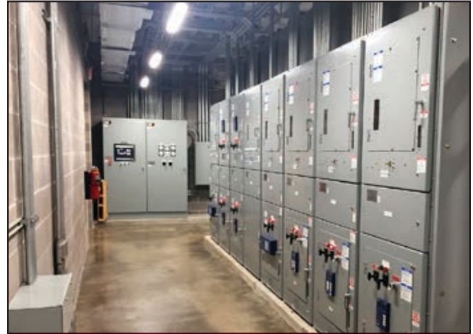
Springdale Water Utilities WWTF Generator Improvements Springdale, Arkansas
