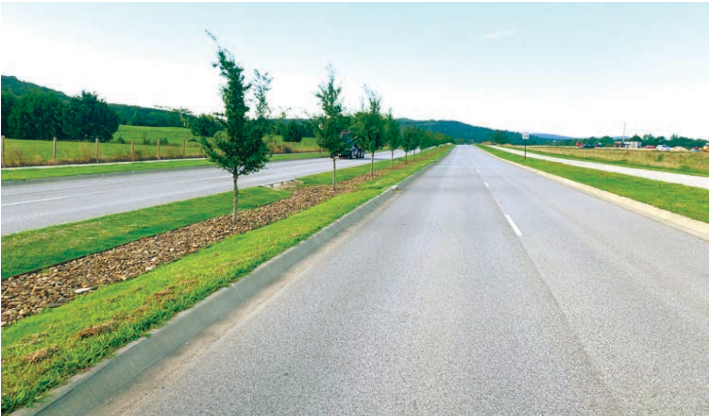
PHOTOS COURTESY MCCLELLAND CONSULTING ENGINEERS
