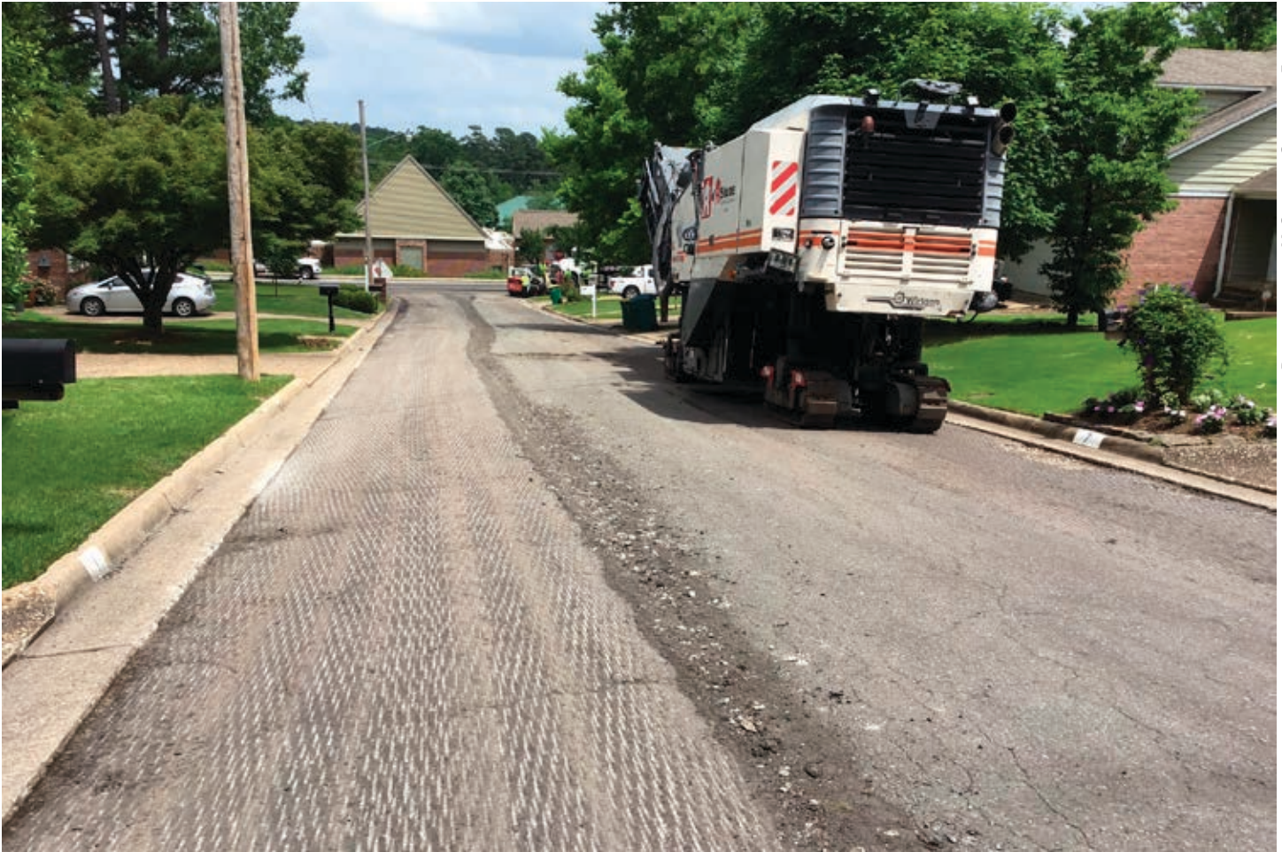
PHOTOS COURTESY MCCLELLAND CONSULTING ENGINEERS
