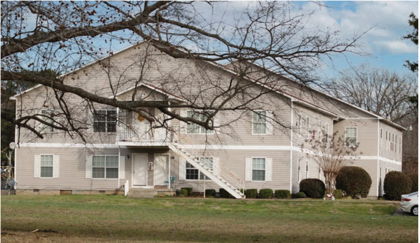
Modular housing? Phil Watkins, Searcy plan/review inspector, remembers this building as delivered in sections that were assembled on-site.
