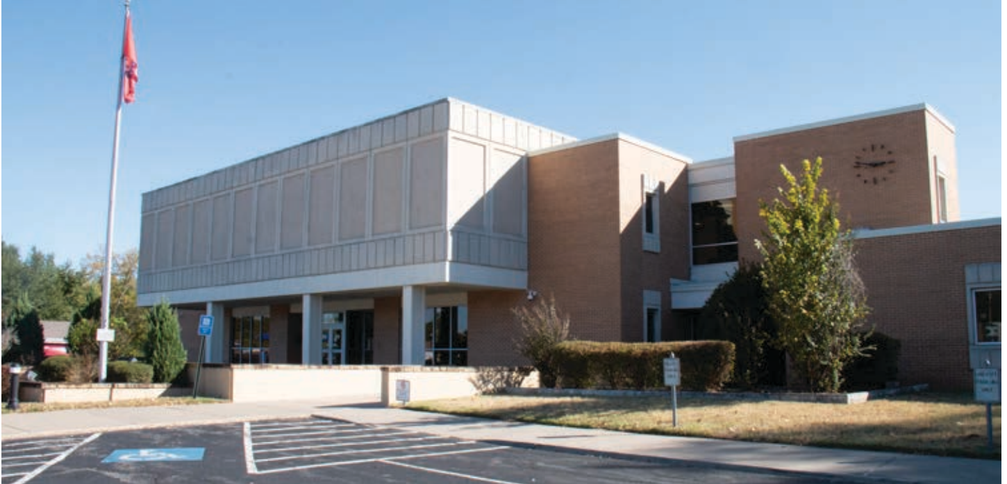
Greenwood is home to one of two Sebastian County courthouses. In a unique jurisdictional designation dating back to the late 19th century, Greenwood is the county seat of lower Sebastian County, while the much larger city of Fort Smith is the seat of upper Sebastian County.
