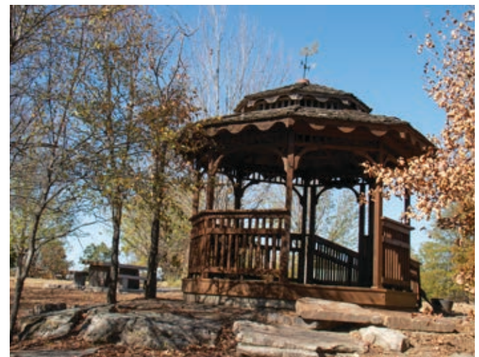
Kinslow calls the 36-acre Bell Park the “crown jewel” of Greenwood’s growing park and trail system. This pavilion and the concrete picnic table beside it are both dedicated to the memories of his parents, Bo and Fred, who loved and supported their hometown.
