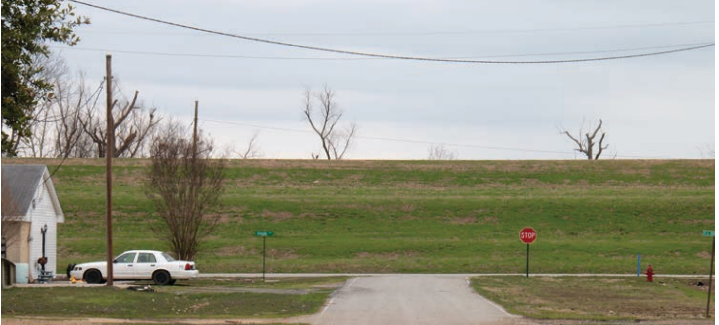
A view of the levee from Capitol Street in Arkansas City.
